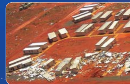
Cyclone George flattens many Port Hedland mining camps in March 2007. NO Screw piles were used on this site.
